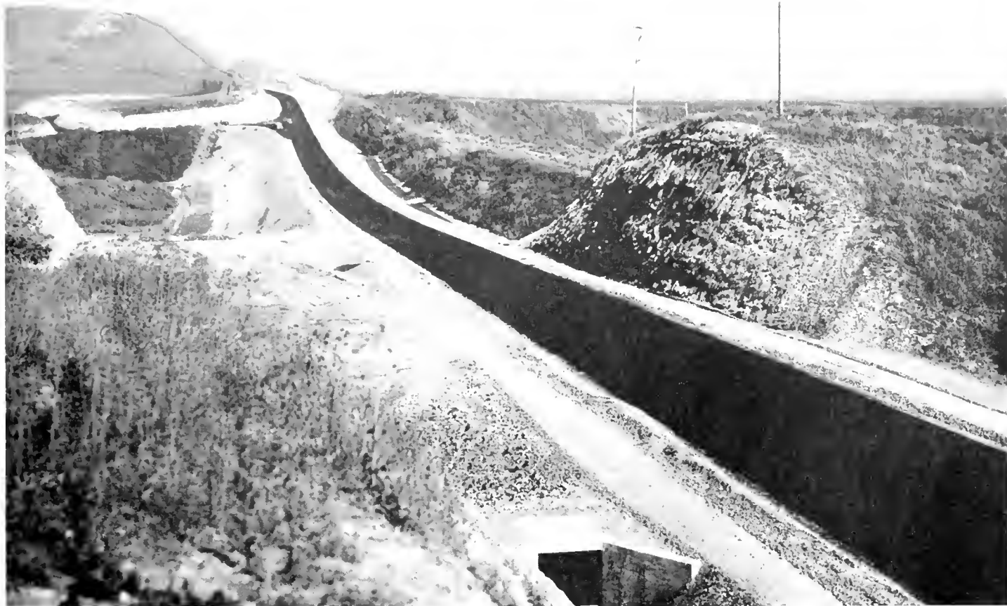
Looking south toward Laguna Creek fill
